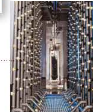
Powder Coat Paint Booth
